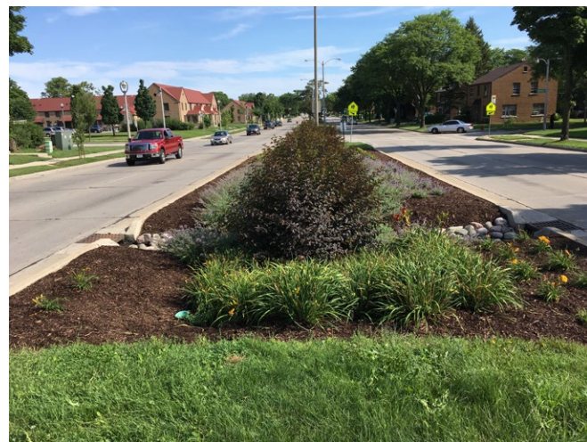
Examples of new bioswales installed by the City of Milwaukee in the median of S. 27th Street and other major divided thoroughfares throughout the city (City of Milwaukee)
