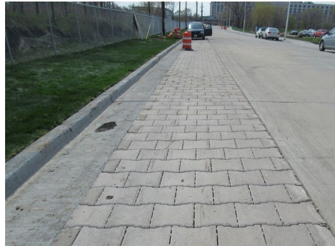
Permeable pavers installed on Greenfield Avenue near the School of Freshwater Sciences (City of Milwaukee)
