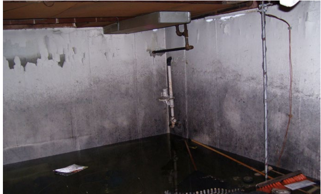
A typical basement backup that could be reduced if green infrastructure strategies are installed in strategic areas within subbasins
