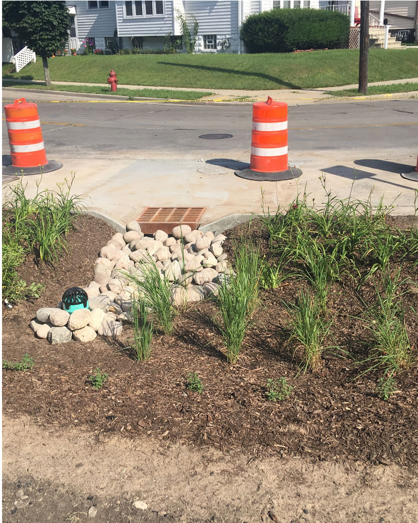
Bioswale installed in the neighborhood surrounding Pulaski Park
