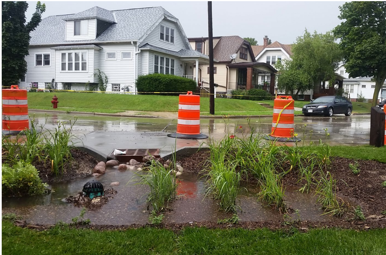
A new bioswale installed in 2017 near Pulaski Park
