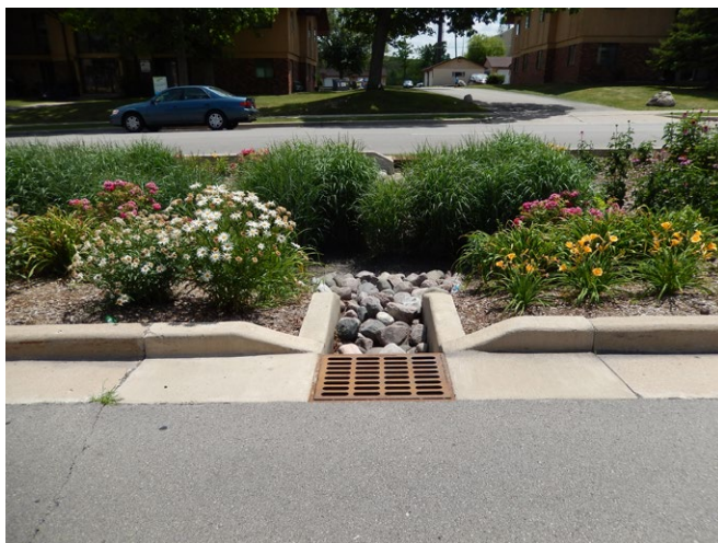
Examples of new bioswales installed by the City of Milwaukee in the median of S. 27th Street and other major divided thoroughfares throughout the city (City of Milwaukee)
